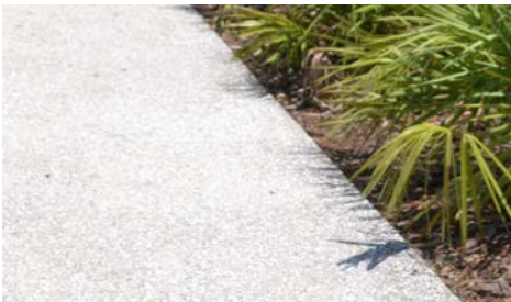
EXPOSED AGGREGATE CONCRETE
