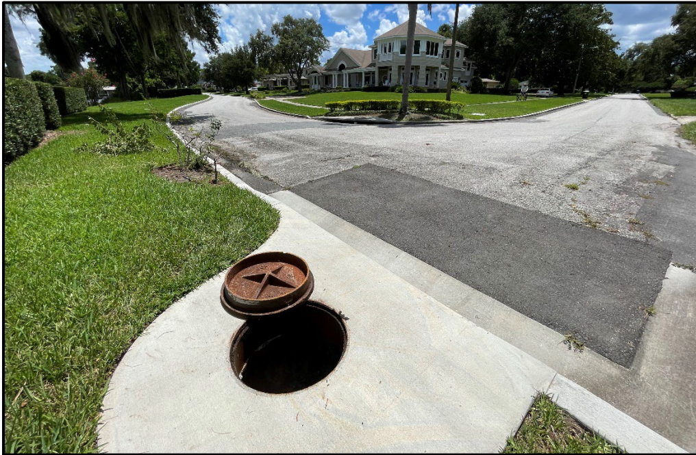
Photograph 4: Site conditions and existing drainage infrastructure at the east end of Euston Road
