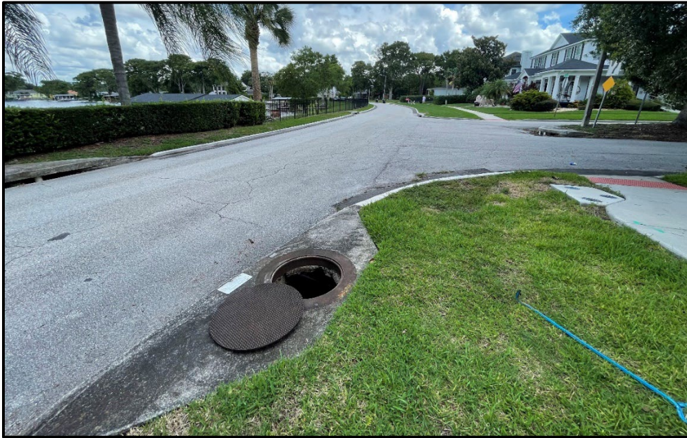
Photograph 8: Existing drainage infrastructure at the intersection of Killarney Drive and Salisbury Boulevard
