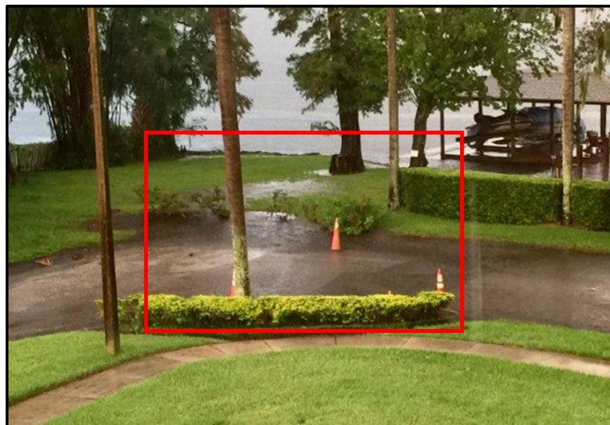
Photograph 1: Flooding and roadway overtopping at the east end of Euston Road
