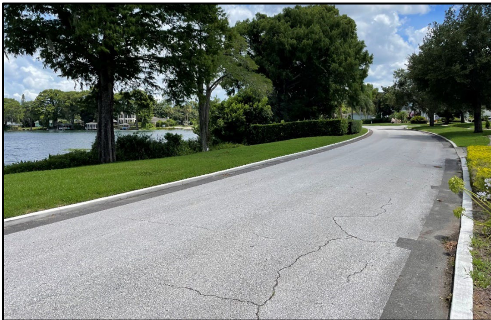
Photograph 7: Site conditions looking south along Killarney Drive
