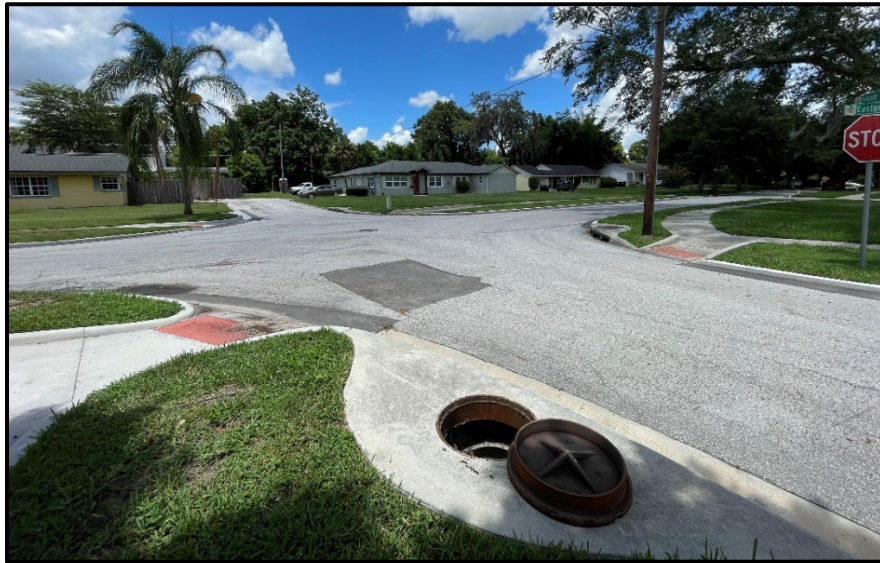
Photograph 2: Existing drainage infrastructure at the intersection of Pelham Road and Euston Road
