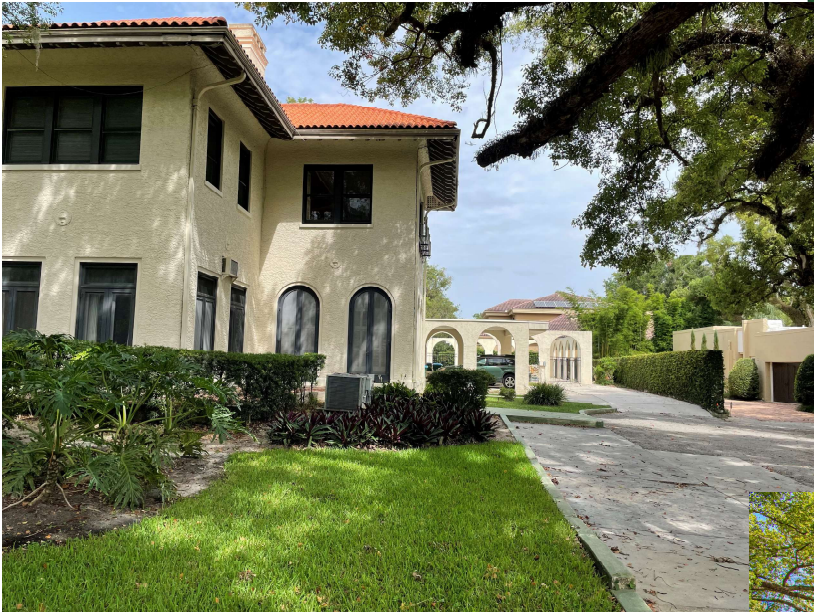
Existing view facing East toward proposed garage location
