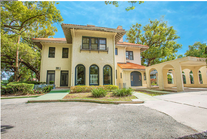
Existing view facing North towards existing mudroom & carport
