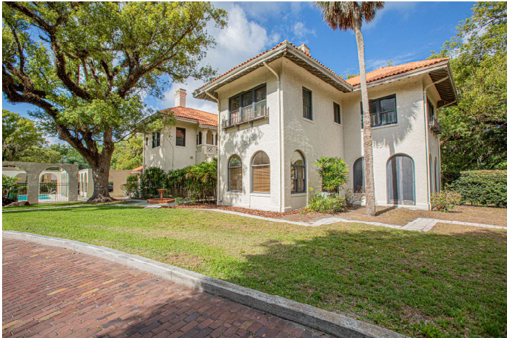
Existing view facing South towards existing Pool and backyard
