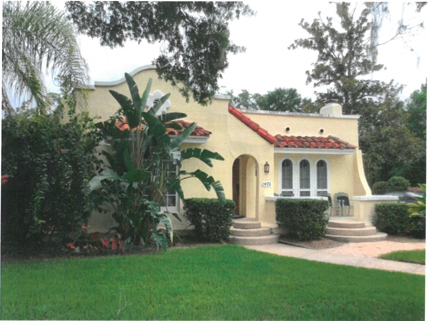
1475 BERKSHIRE AVE, WINTER PARK, FL 32789 6/19/2019 10:13 AM
