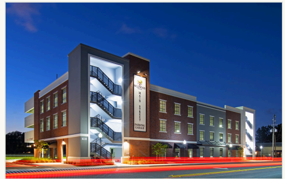
WILDWOOD PARKING GARAGE — DELIVERED 2024, P3 WITH G3
