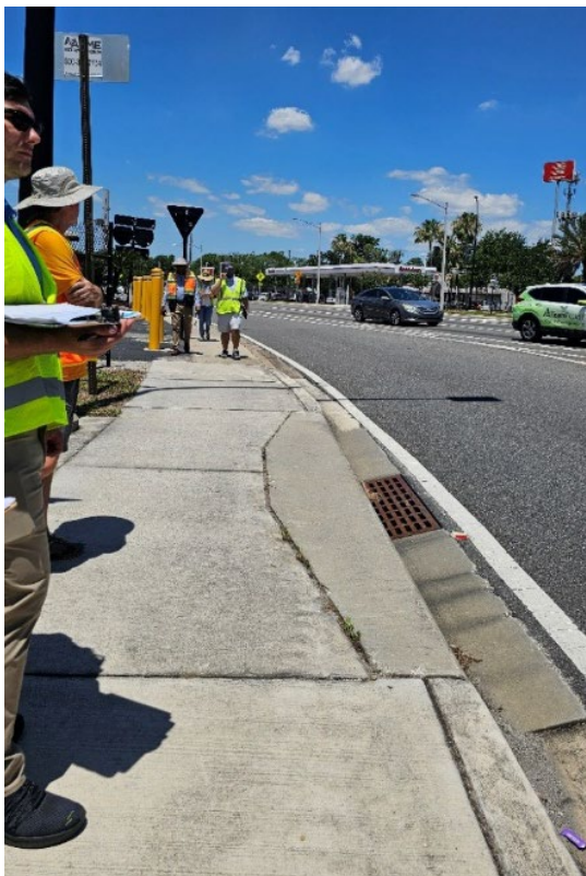
Curve of roadway creates poor sightlines for pedestrians at southwest crossing, before Interstate 4
