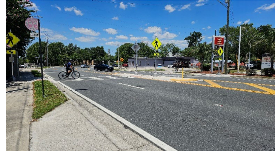
Recently installed RRFB between Driver Avenue and Overspin Avenue can improve crossing options and safety
