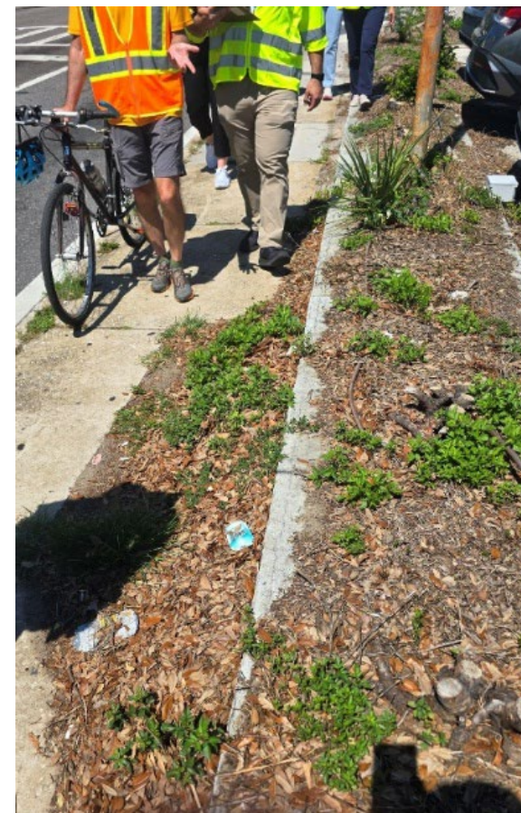
Narrow sidewalks with significant vegetation debris limiting pedestrian access at the North sidewalk on the SR 426 in front of Holler Honda looking west
