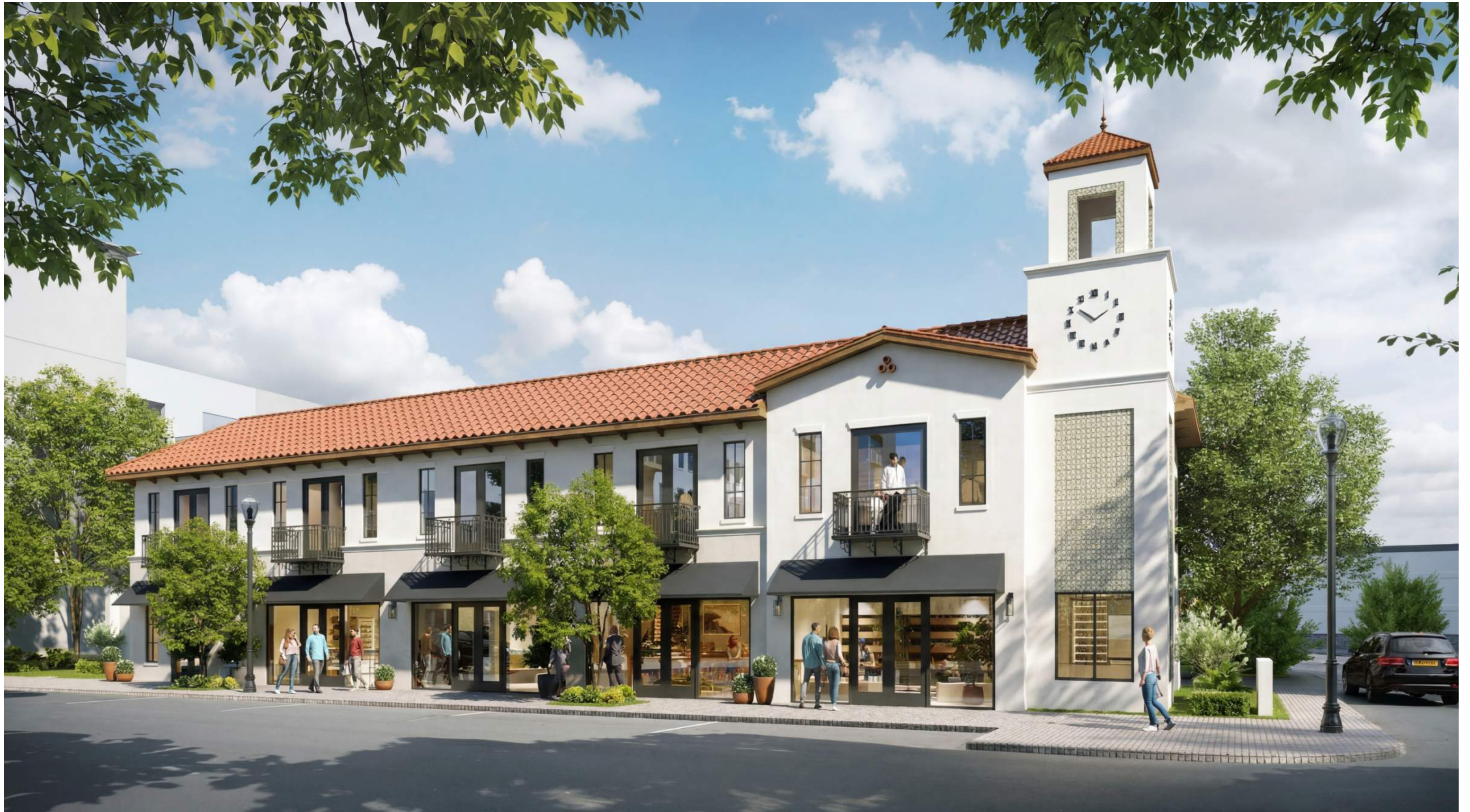
RAVAUDAGE WINTER PARK 1006 LEWIS DRIVE, WINTER PARK MXU BLDG DRC APPLICATION PACKAGE
