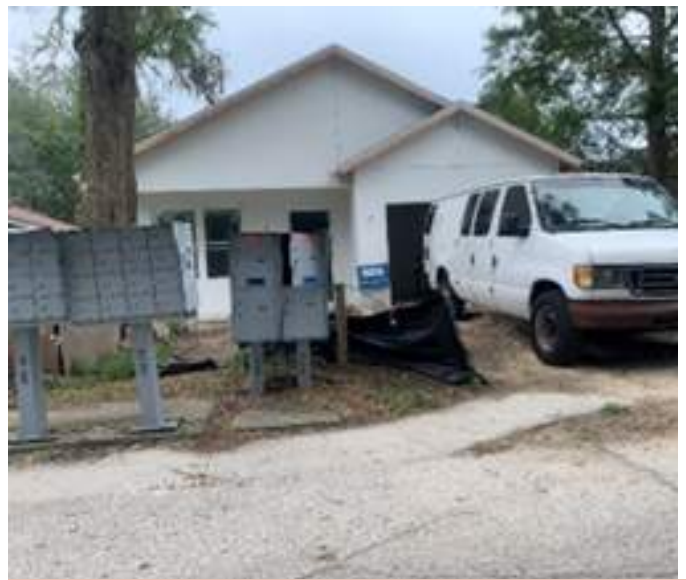
Deteriorated group mailboxes.
