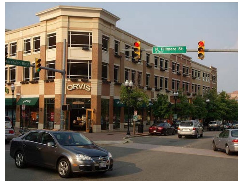
The photo above shows a parking garage seamlessly integrated into the landscape with retail on the ground floor that serves to activate the entire block.
