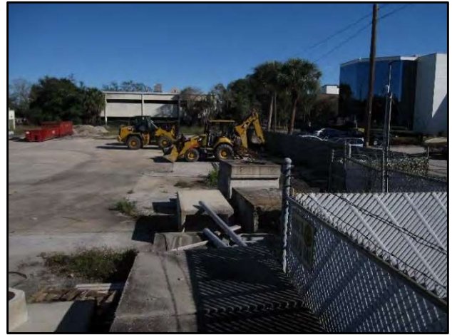
View east from near the subject's and Parcel A's southwest corner
