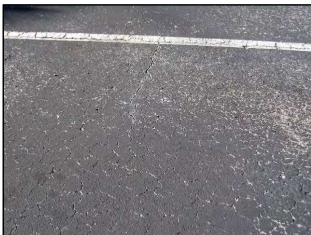
Parcel C's asphalt paved parking totals 52 spaces in fair to average condition (cracked but sealed).
