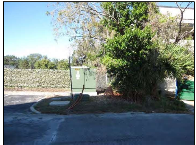
The subject's approximately 19' frontage on W Swoope Ave is obstructed by an electric transformer recently installed in the right-of-way.
