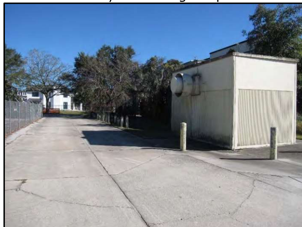
In addition to the driveway (at left), the access strip hosts a pump house for the city's nearby water plant and a small retention pond.
