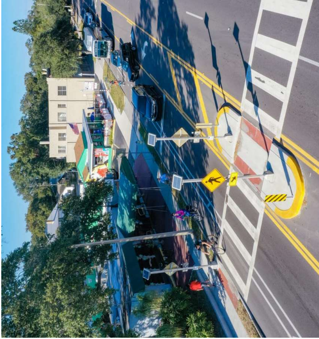
Lane re-allocation to install buffered bike lanes & enhanced crossing as part of resurfacing project in St. Petersburg, FL - Dr. MLK Jr. Street
