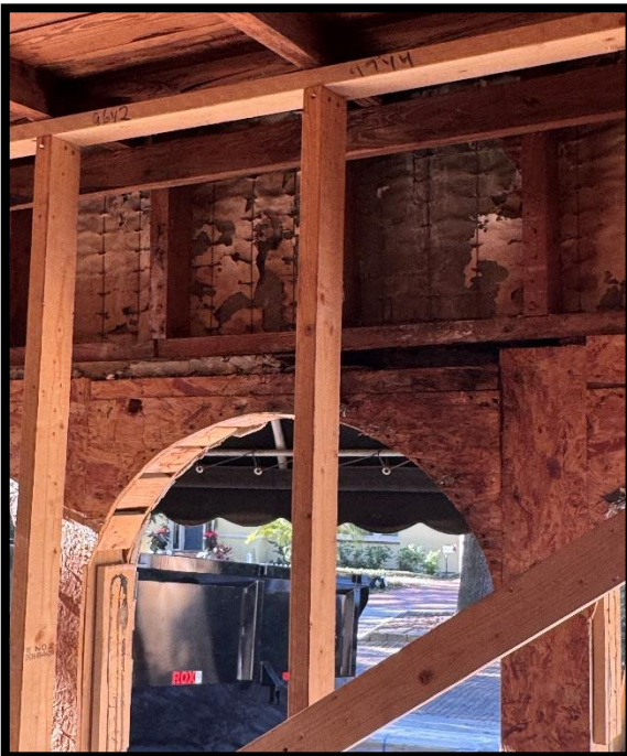
These photos indicate the compromised top of wall, WDO infestation, and water intrusion.
