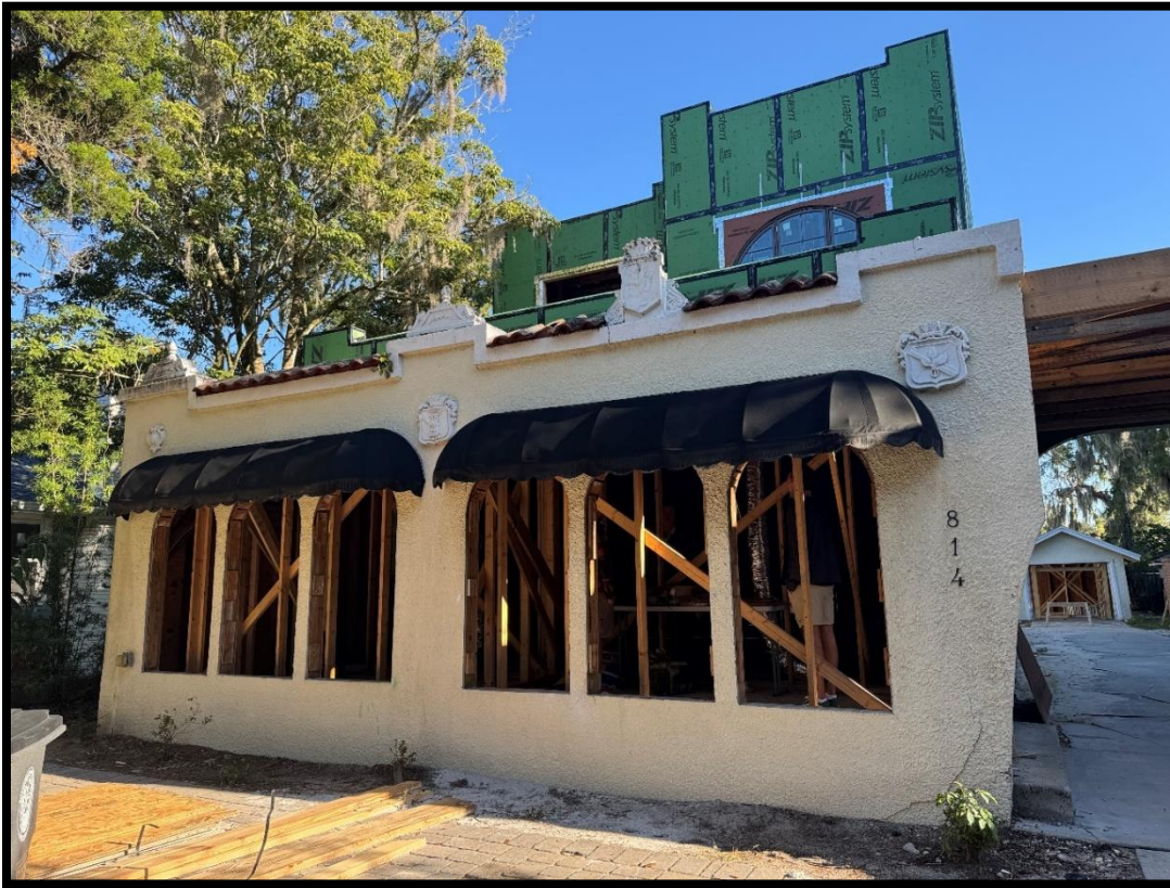
These openings shown in the picture above are not original to the home and were repaired at some point in the past.
