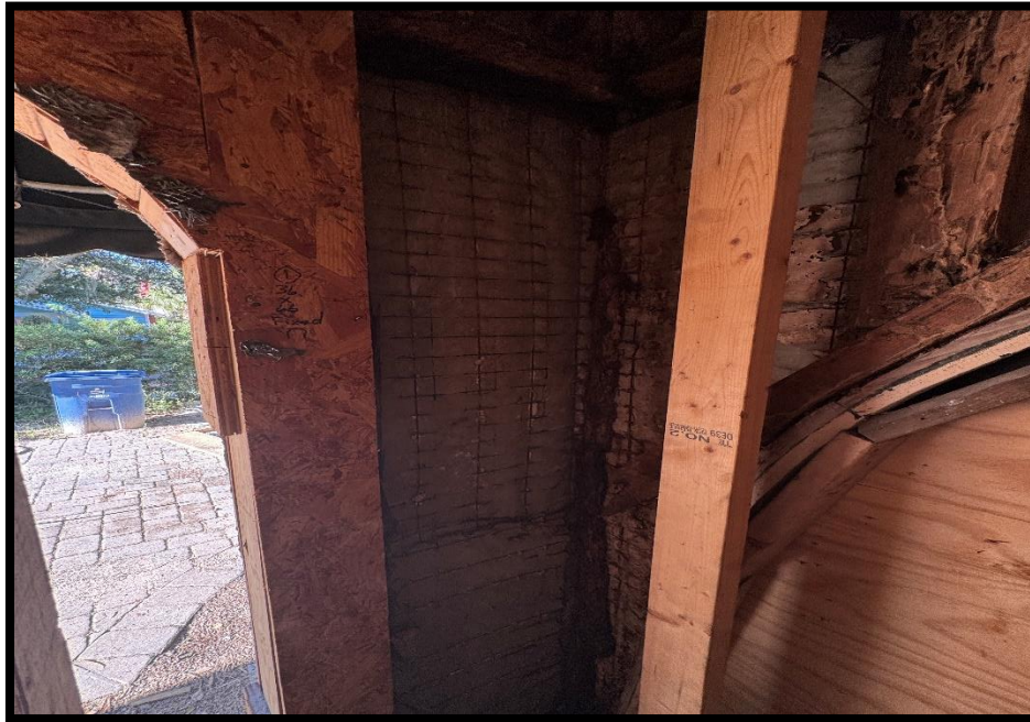
This photo indicates no structural components exist.
