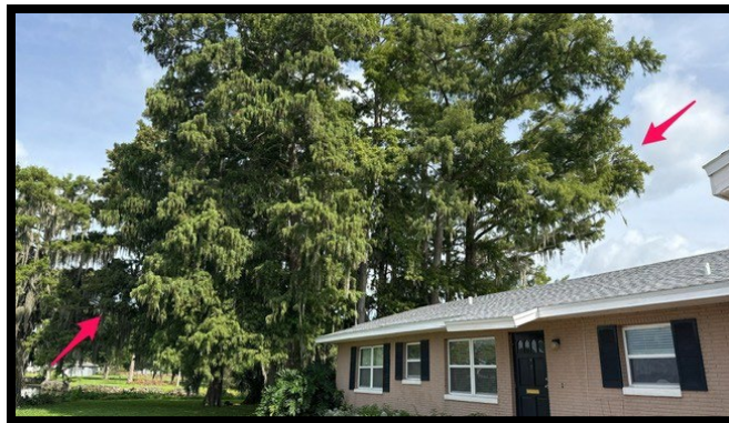
Heavy canopies over existing structure
