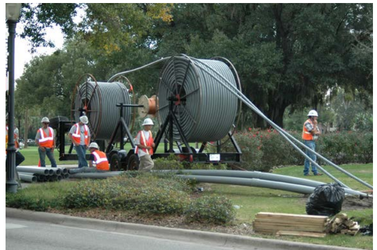
Crews conducting undergrounding work. Photo courtesy City of Winter Park.
