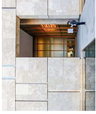
The Barnes Foundation, Philadelphia, PA Contemporary Stone Facade
