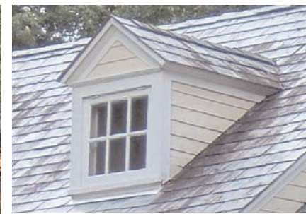
Colonial Revival style dormer
