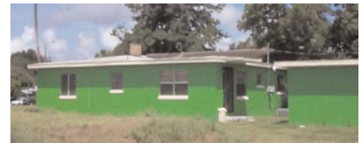
Inappropriate Colors for a Historic District
