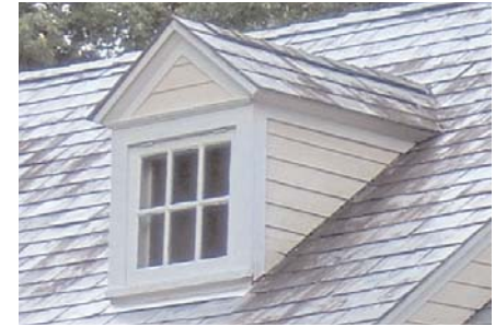
Colonial Revival style dormer
