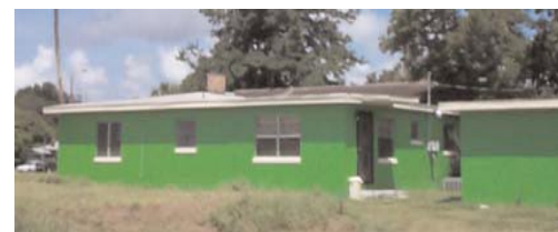
Inappropriate Colors for a Historic District
