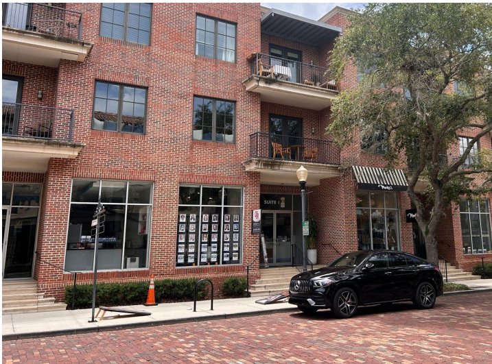
Terrace with recessed entry
