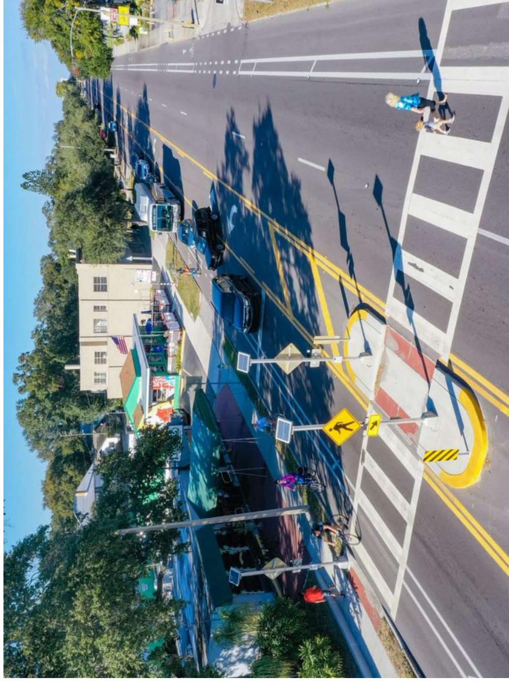
Lane re-allocation to install buffered bike lanes & enhanced crossing as part of resurfacing project in St. Petersburg, FL - Dr. MLK Jr. Street at 13 th Avenue N
