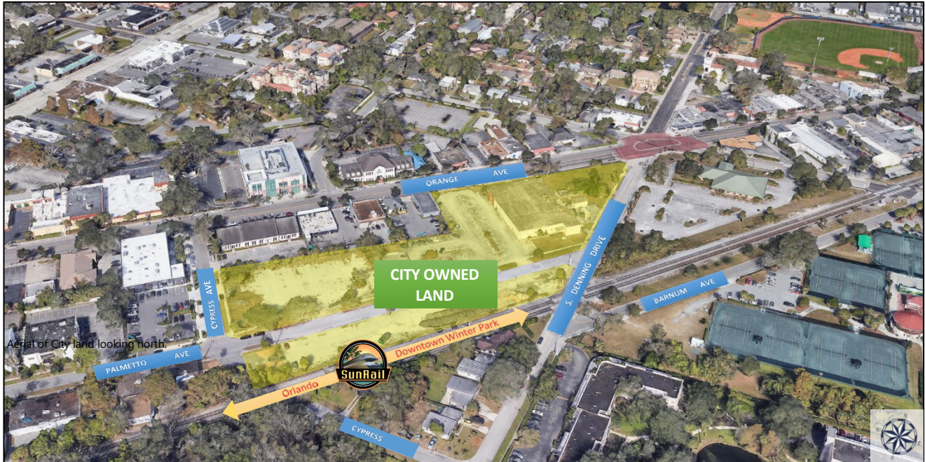
Aerial of City Owned Land looking north.
