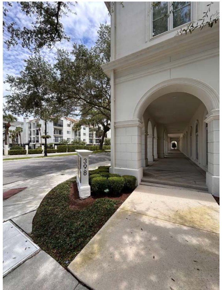
Gallery with enhanced hardscape.
