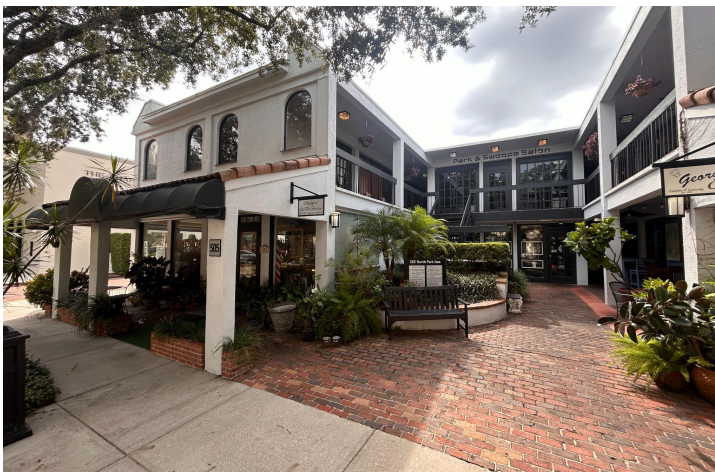
Gallery with a forecourt and cafe seating
