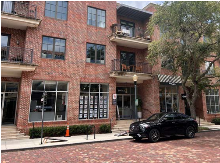
Terrace with recessed entry
