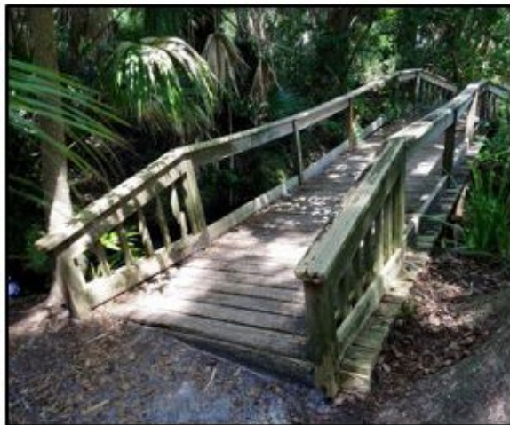
Figure 3-1. Mead Botanical Garden pedestrian bridges
