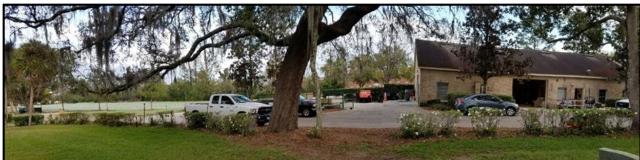
Figure 3-4. Existing building shared by Palm Cemetery and golf course maintenance.
