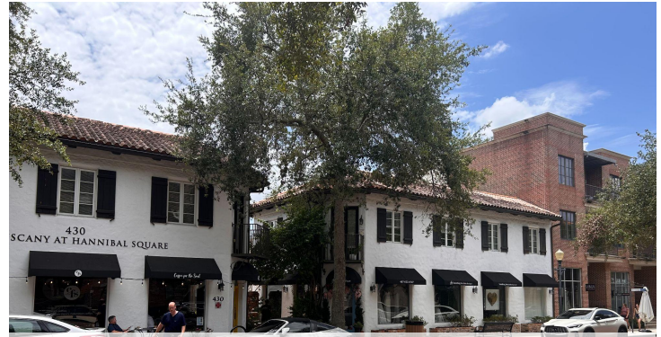
In this image the ground floor transparency is higher than the upper floors, the shutter and awning colors are coordinated and the interior courtyard creates a meaning articulation in the building.
