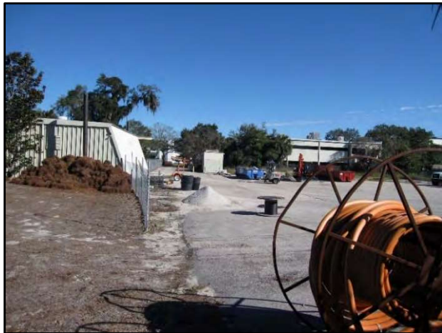
View east from subject's northwest corner along north property line
