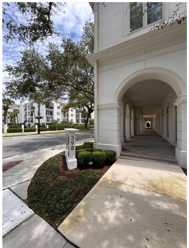
Gallery with enhanced hardscape.
