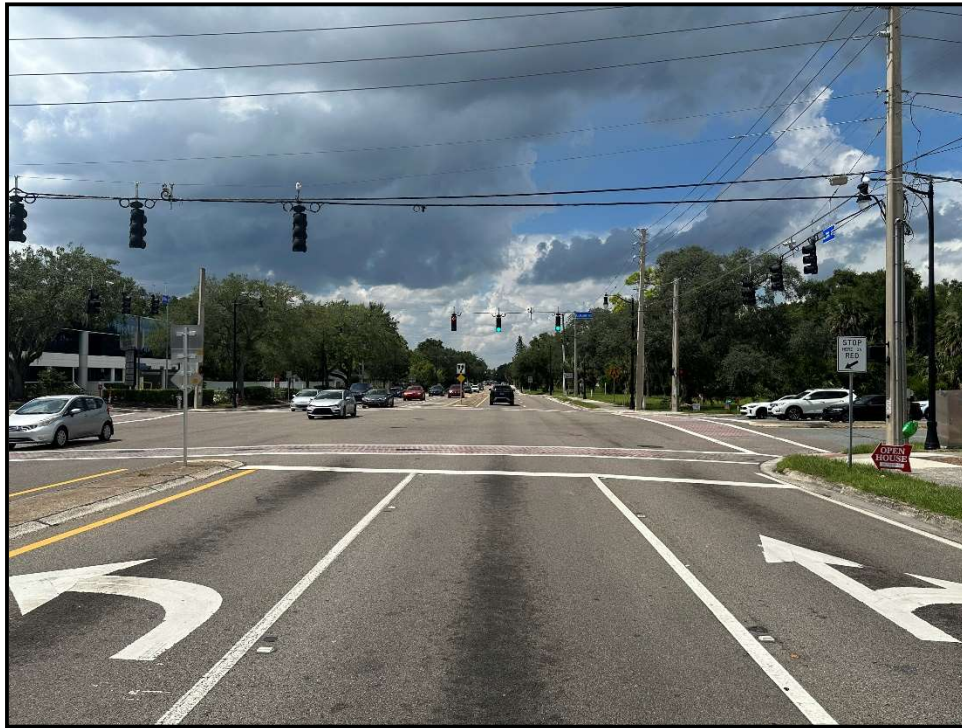
Looking West Toward Intersection
