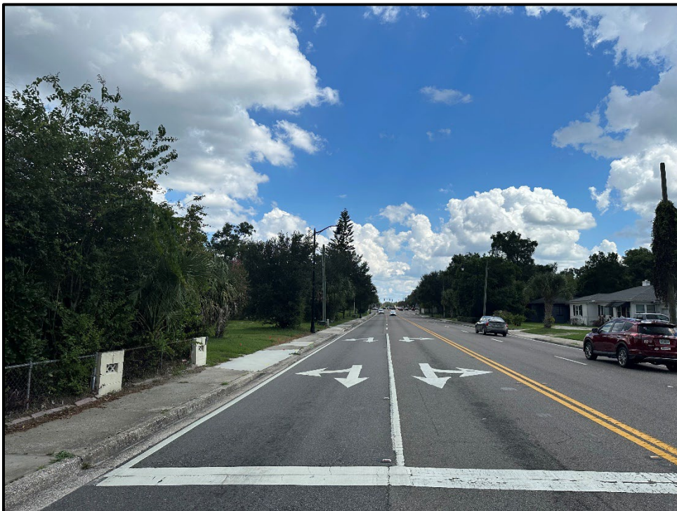
Looking East Away from Intersection
