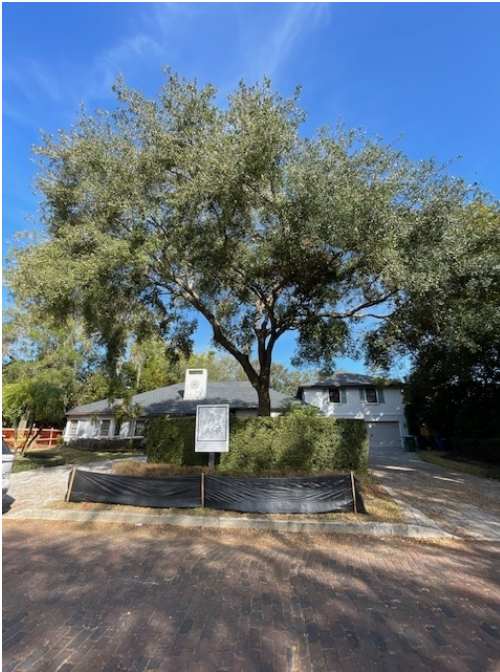
Live oak 23" No notable defects
