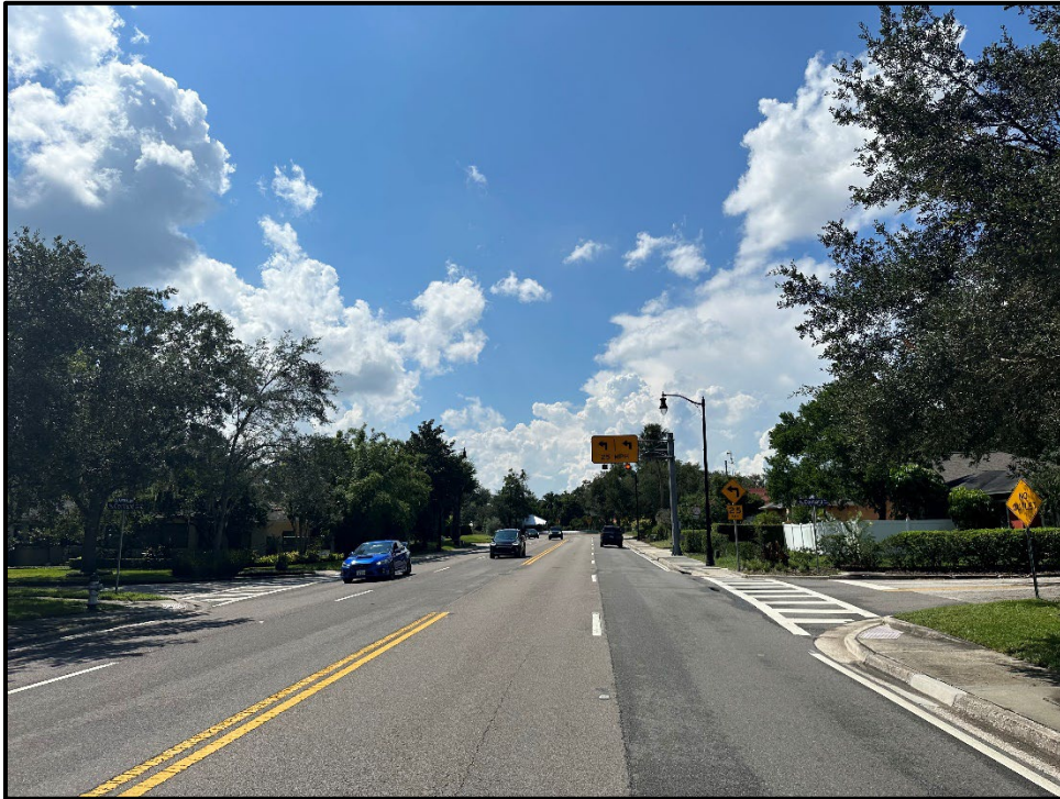
Looking West Toward Intersection
