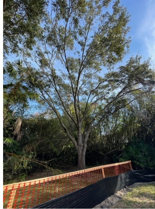
Live oak 22" Notable Defect: • Low codominant stem, usually not an issue for live oaks
