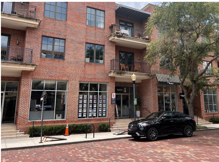
Terrace with recessed entry
