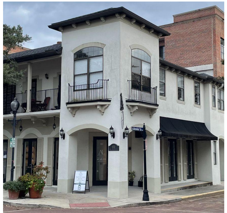
Brackets and Corbels – Decorative supports under eaves or ledges, often carved or shaped.
