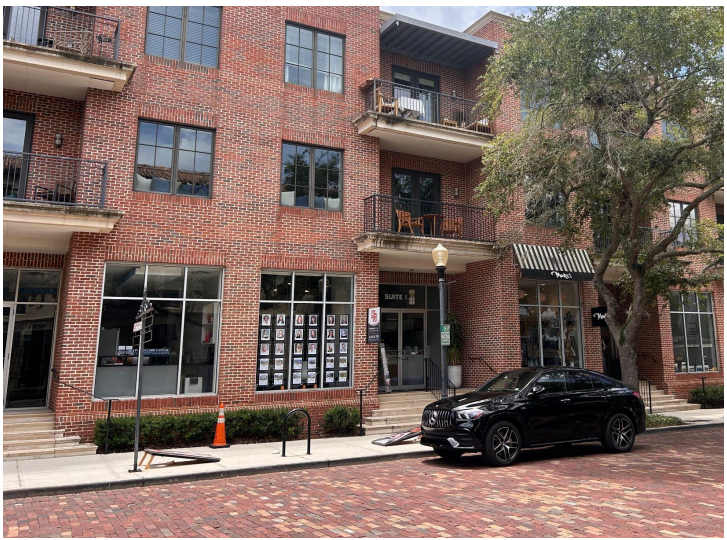
Terrace with recessed entry
