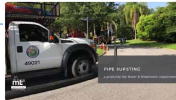
Water Pipe Installation - Pipe Bursting
