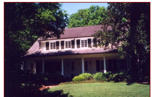
Plate 22. Webster House, 461 Webster Avenue
