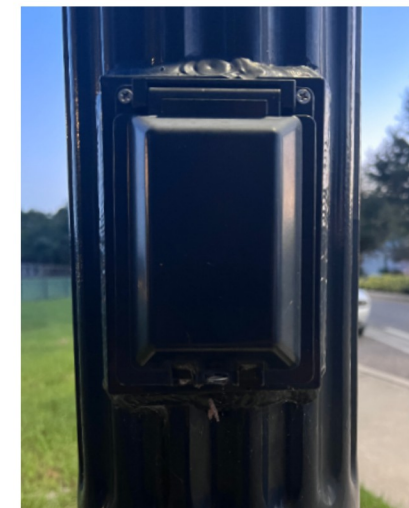
Existing light pole for reference
