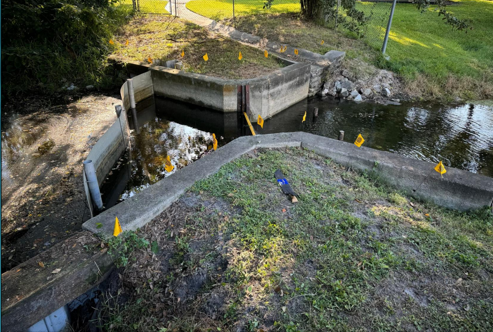
Lake Bell Weir Repair
