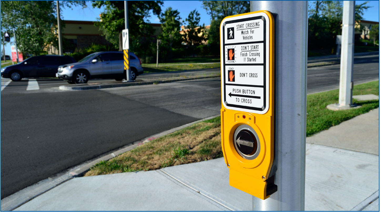
Figure 10 - Accessible Pedestrian Signal (APS) push buttons. ( https://commons.wikimedia.org/wiki/File:PedestrianSignalPushButton.jpg )
