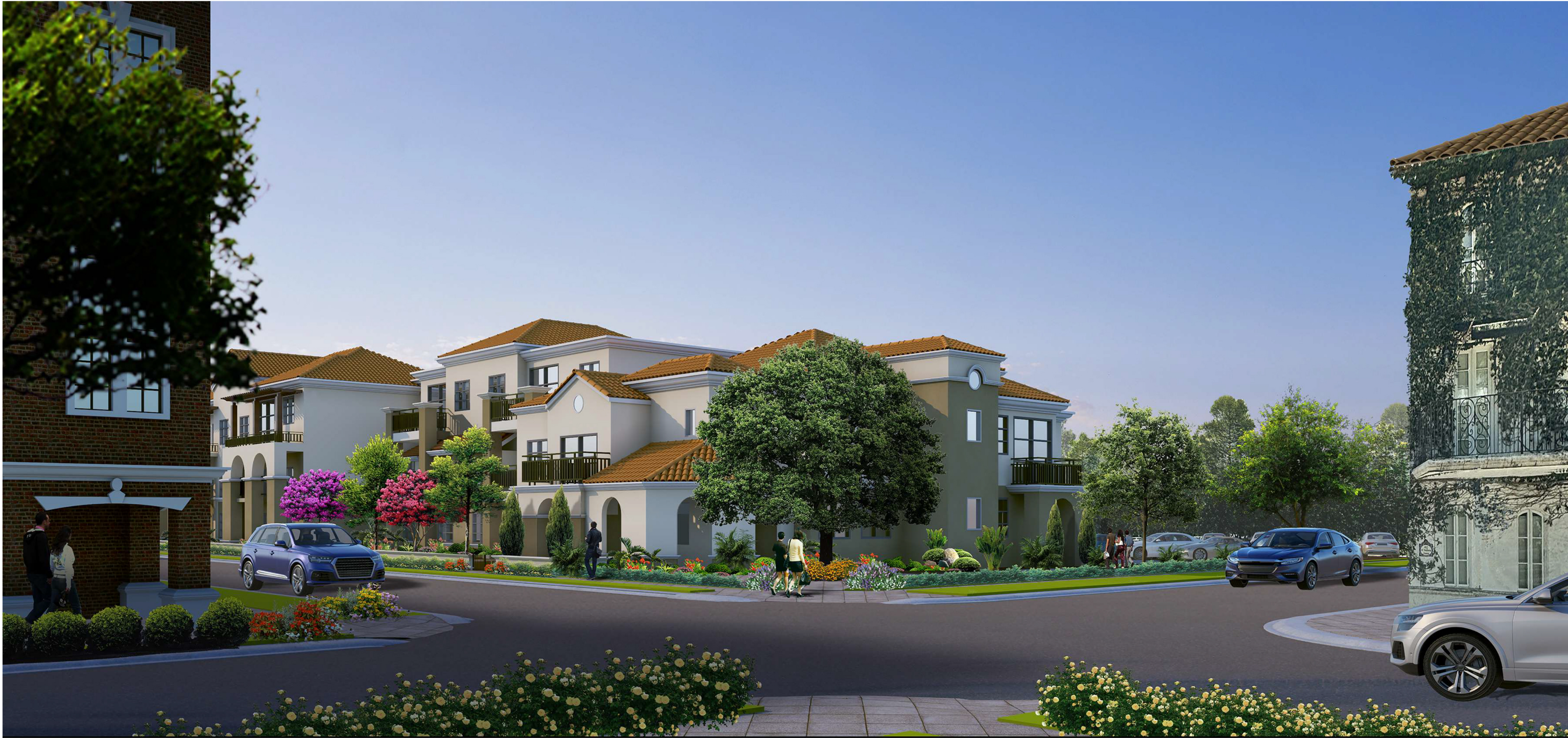
VIEW FROM WELBOURNE AND VIRGINIA
