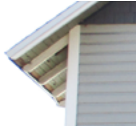
Exposed Rafter Tail
