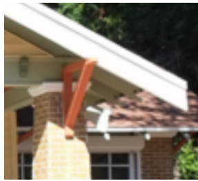
Exposed Rafter Tail
