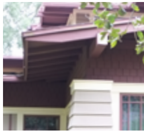
Exposed Rafter Tail
