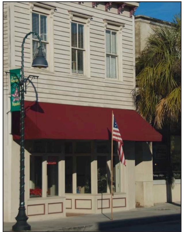
Shopfront with formal window frames and bracketed cornice
