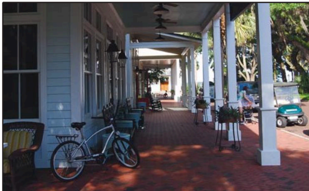
Gallery and double-hung windows on commercial building
