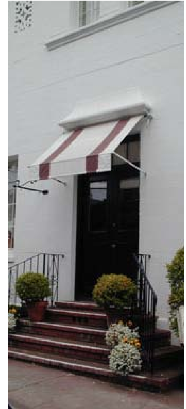
AWNINGS FIT IN OPENING WITH VALANCE
