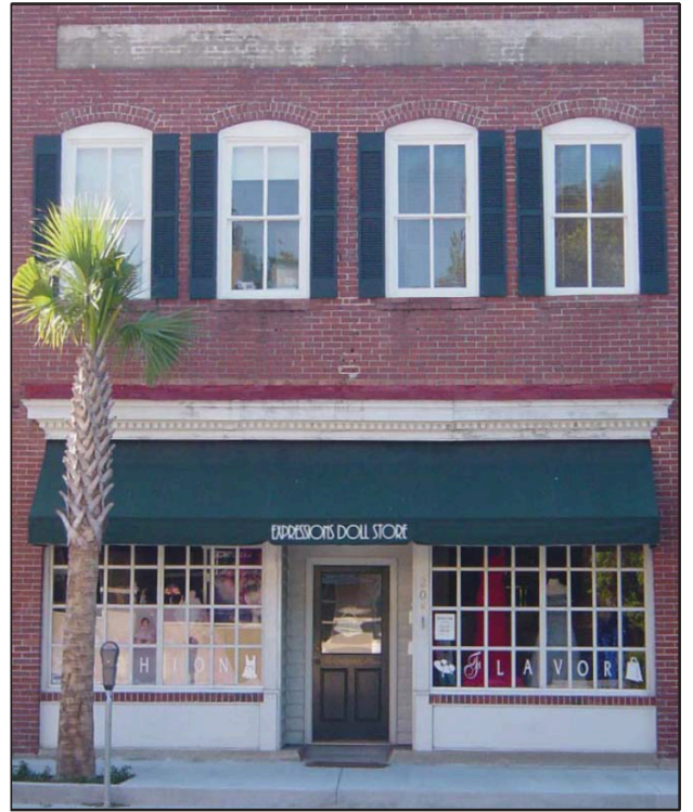
Shopfront with classical dentils and divided lights
