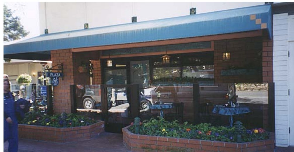
LONG, HORIZONTAL AWNINGS NOT ALLOWED
