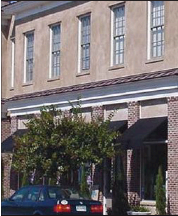
Stucco building with brick piers
