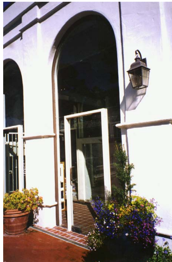
SHIELDED LIGHT FIXTURE
