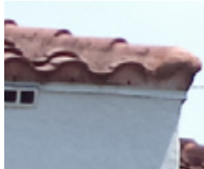
Minimal Eave Overhang
