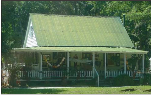
Steep-sloped roof and porch on a residential-form building
