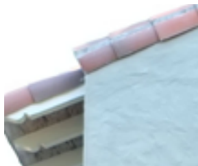
Exposed Rafter Tail
