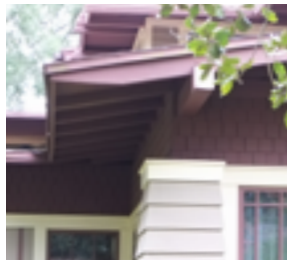
Exposed Rafter Tail
