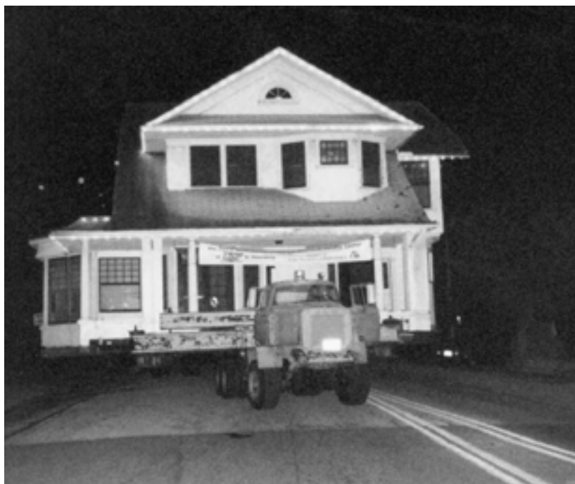
Overnight relocation of the Snell House to the University of South Florida St. Petersburg Campus August 1993.
