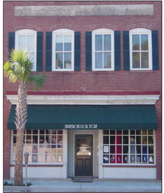
Shopfront with classical dentils and divided lights
