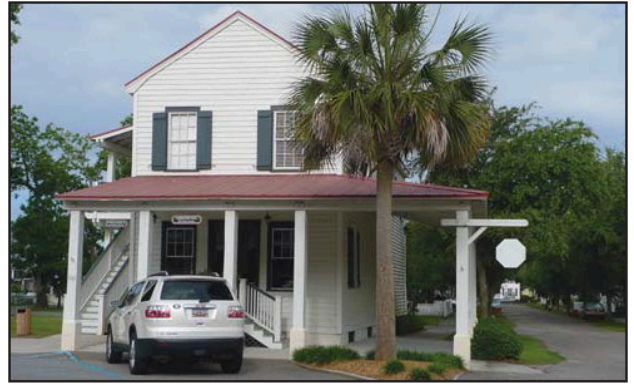
Wood siding and simple gable form on a commercial building
