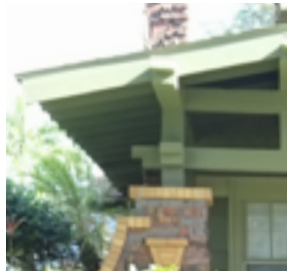
Exposed Rafter Tail
