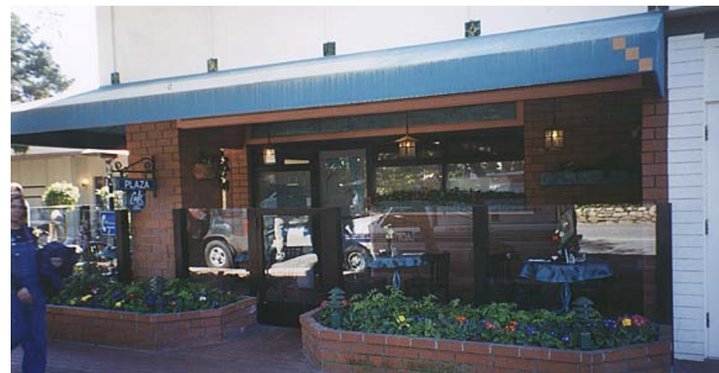
LONG, HORIZONTAL AWNINGS NOT ALLOWED
