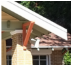
Exposed Rafter Tail
