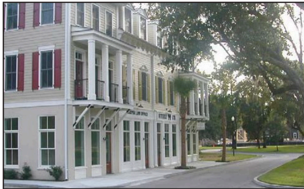
Balconies with wood brackets
