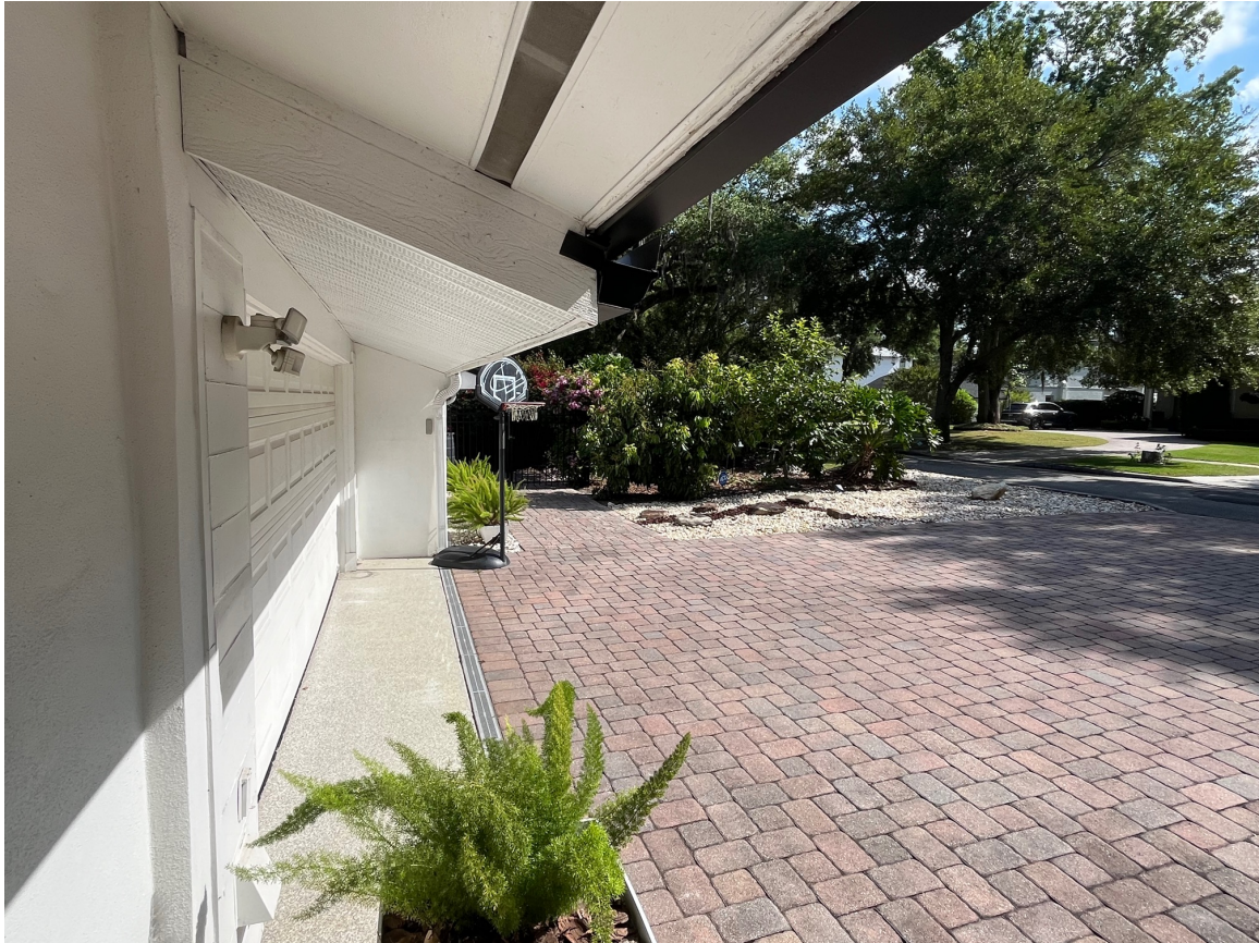
North View (facing 1252 Via Del Mar)
