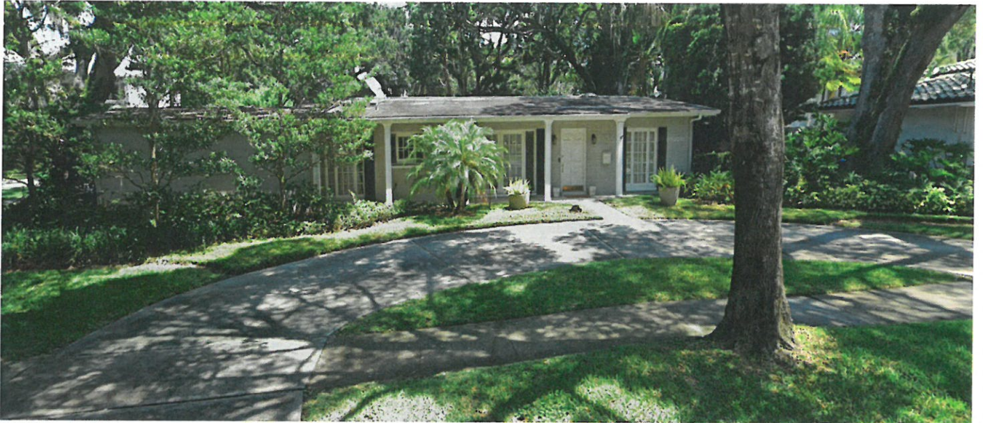
View of Existing Home from Stirling Avenue
