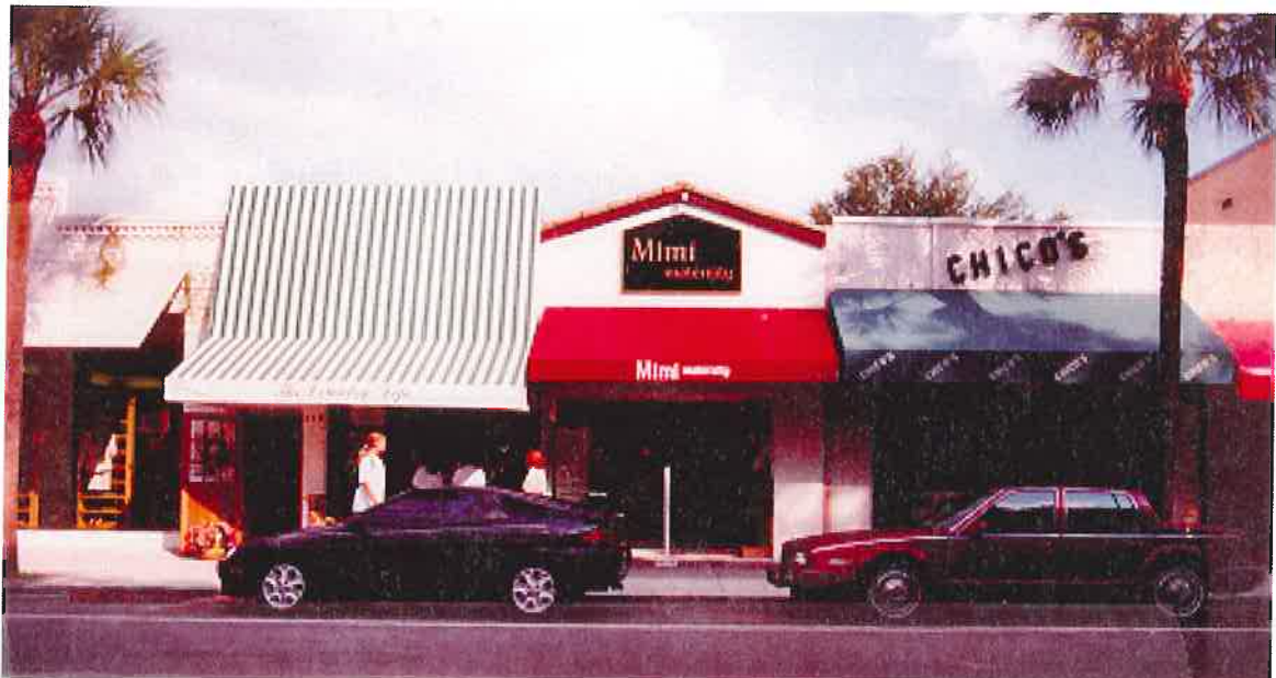
Awning with Green Stripes too Large for Building
