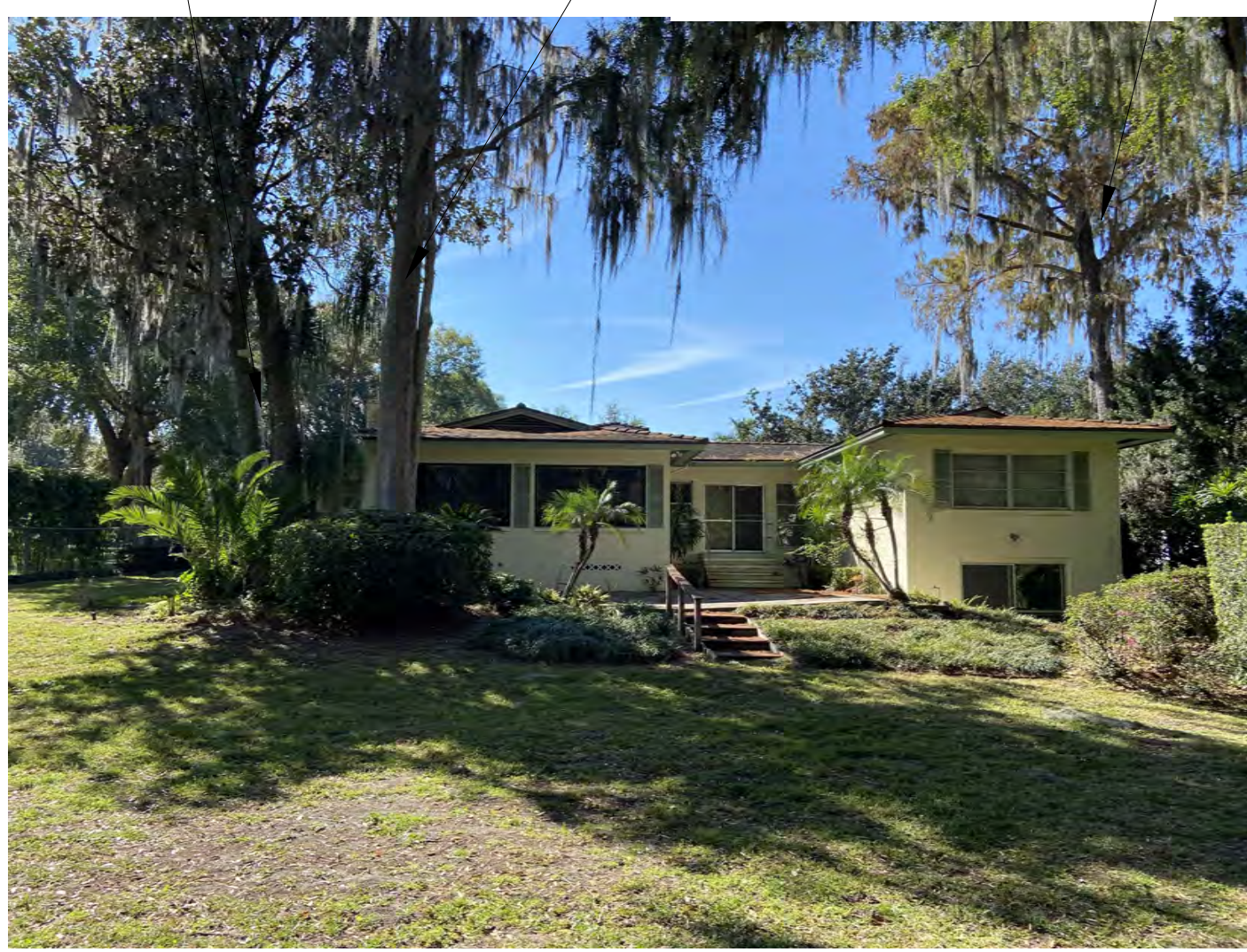
PIC 2 - VIEW FROM HOWELL CREEK
