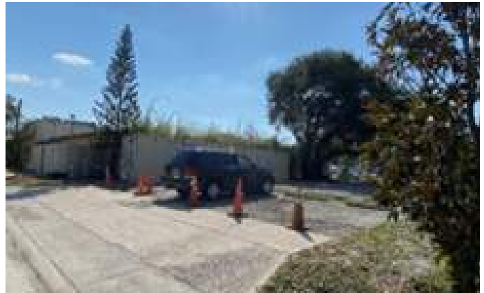
Inadequate and defective parking facilities within the Orlando Avenue Commercial Corridor FON Study Area.
