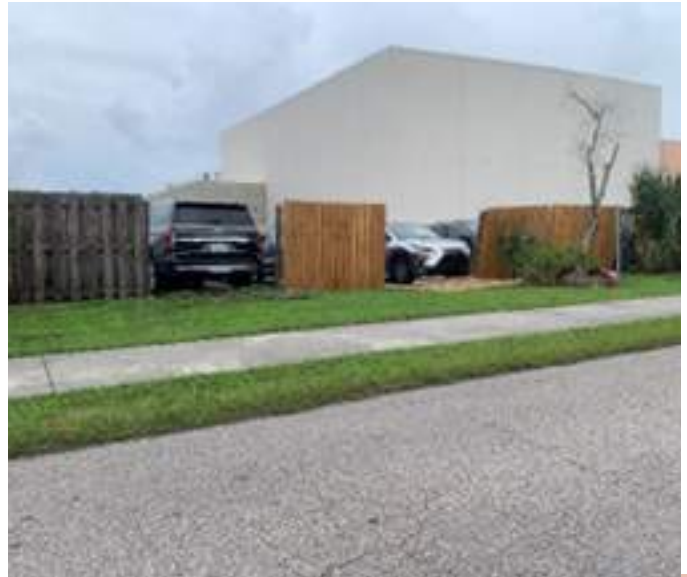
Deteriorated improvements boundary fence.
