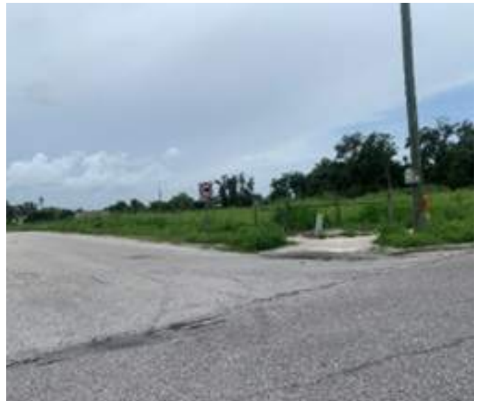
Defective street layout. Sidewalks and roadway serving large undeveloped, superblock, parcels near Rauvadge.
