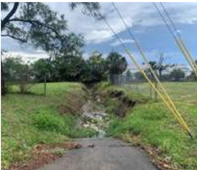
Deteriorated stormwater collection and conveyance improvements.
