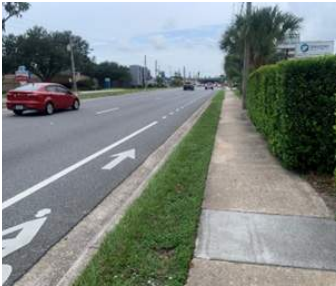
Narrow sidewalks, on-street bike lane and no pedestrian crosswalks to traverse Lee Road.
