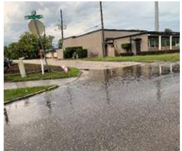
Unsafe and unsanitary conditions from localized roadway flooding & internal parcel flooding within the Fairbanks Avenue FON Study Area.
