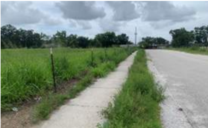
Defective street layout. Sidewalks and roadway serving large undeveloped, superblock, parcels near Ravaudage.
