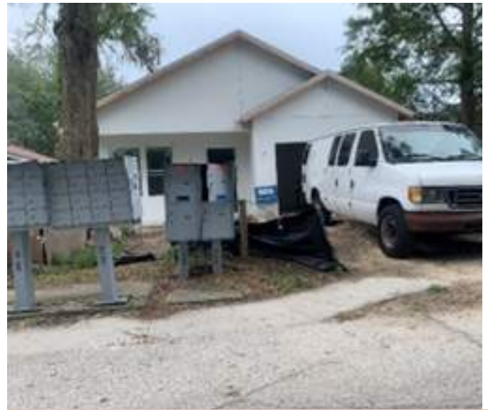
Deteriorated group mailboxes.
