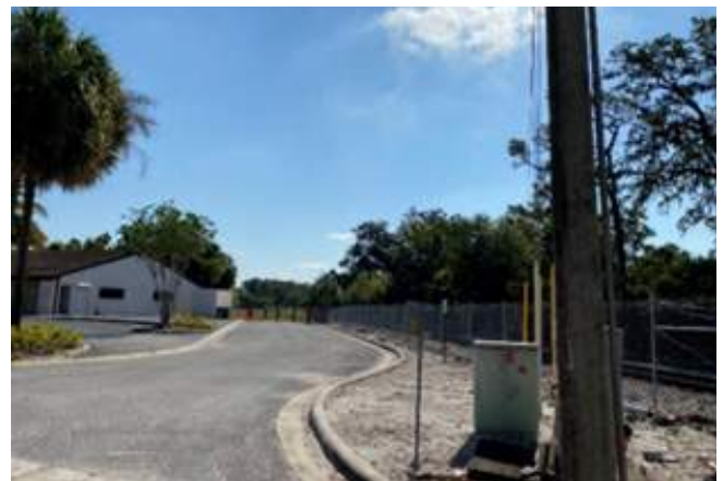
Disjointed and defective roadway layout within the Orlando Avenue Commercial Corridor FON Study Area.
