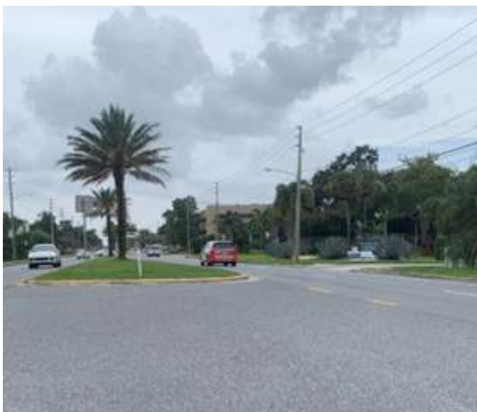
Over 1 mile of 4+ vehicle lanes to cross with no mid-block pedestrian signals, crosswalks, or points of refuge.
