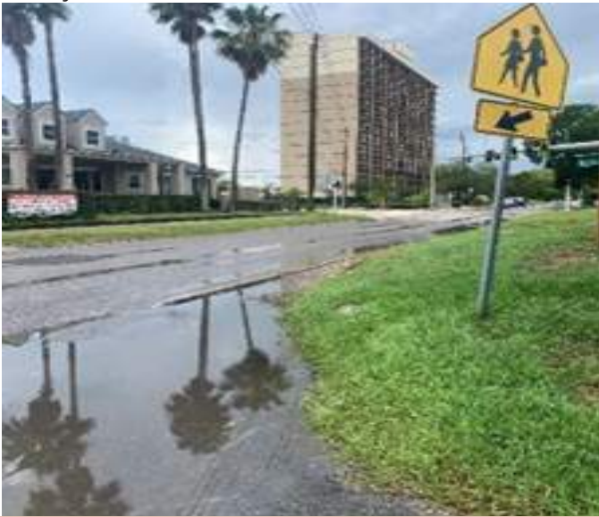
School crosswalk with no sidewalk or crosswalk on lots.
