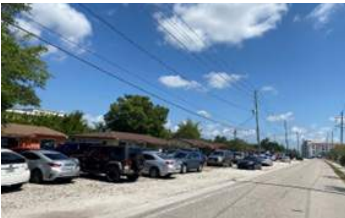
Defective street and parking layout. Cars parking on street frontage, continuous curb-cut.
