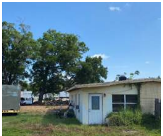
Deteriorated building and site improvements.
