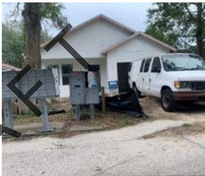
Deteriorated group mailboxes.
