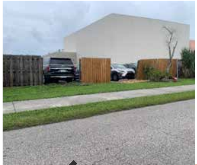
Deteriorated improvements boundary fence.
