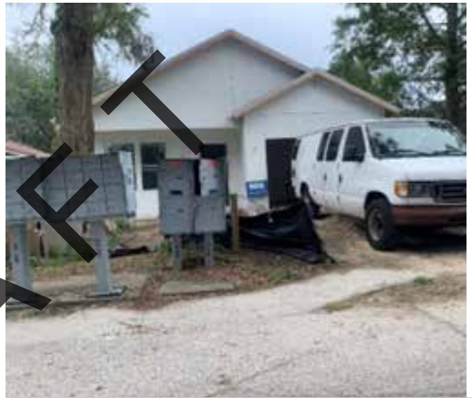
Deteriorated group mailboxes.
