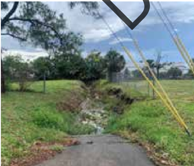
Deteriorated stormwater collection and conveyance improvements.
