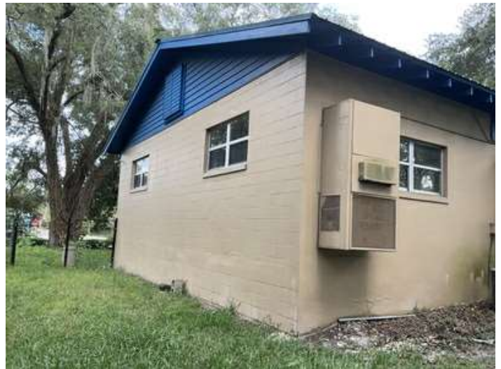
Exterior view of subject
