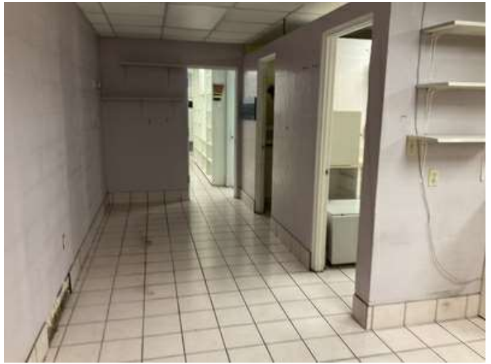
Interior view of subject
