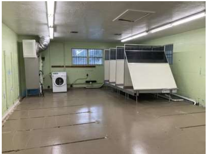
Interior view of subject
