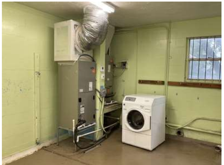
Interior view of subject
