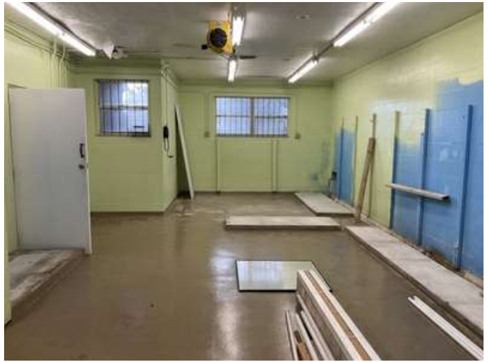
Interior view of subject
