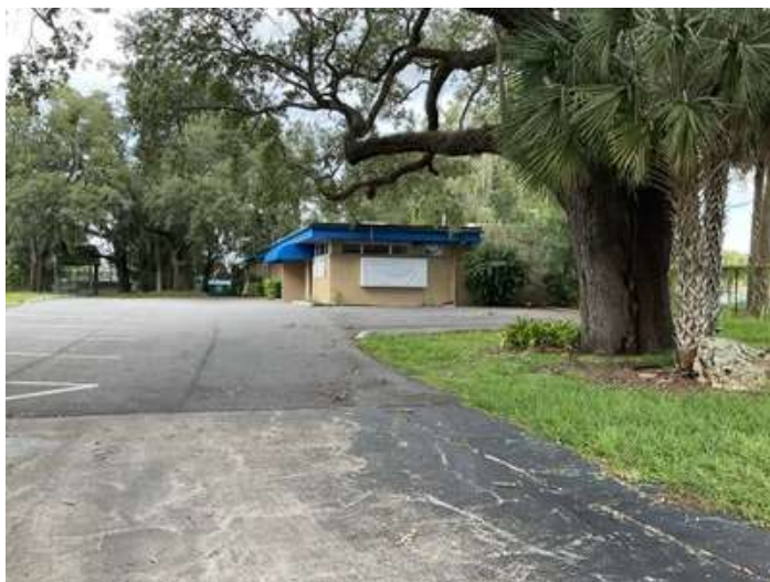
Exterior view of subject
