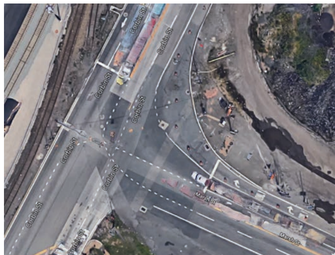
Figure 21. Double right-turn lanes for trucks leaving Port Newark. (Photo source: Google Earth.)
