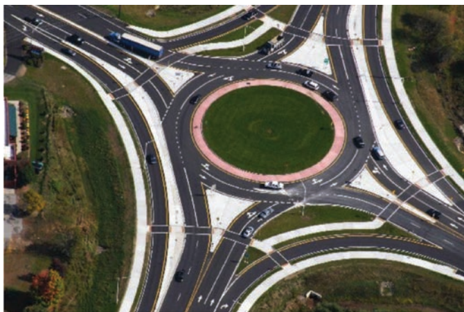
Figure 35. Typical roundabout with right-turn bypass lane. (Photo source: New Hampshire DOT.)
