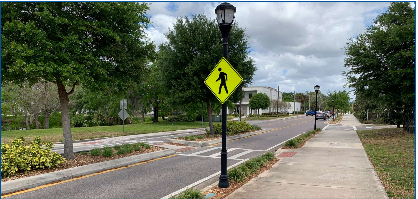
Figure 1 - Denning Drive shared use path and enhanced crossing.
