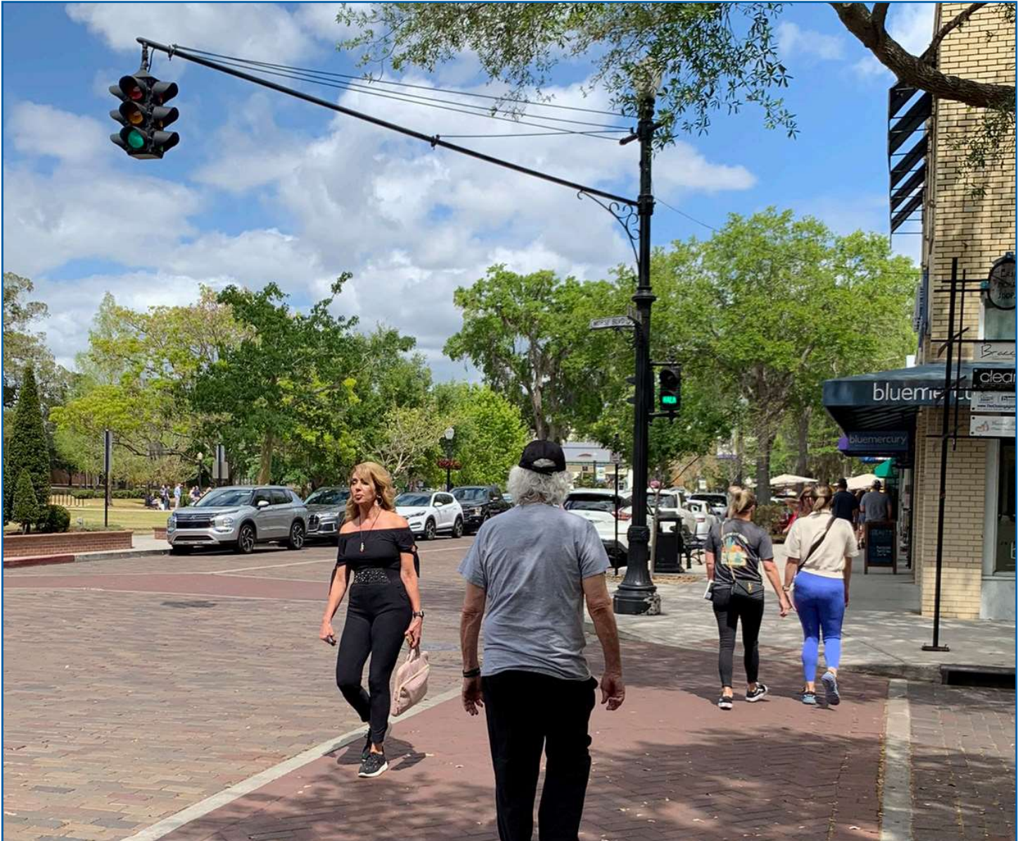
Figure 3 - Legacy traffic signal equipment along Park Avenue
